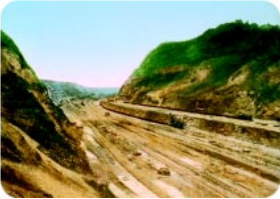
PANAMA CANAL — CULEBRA CUT
